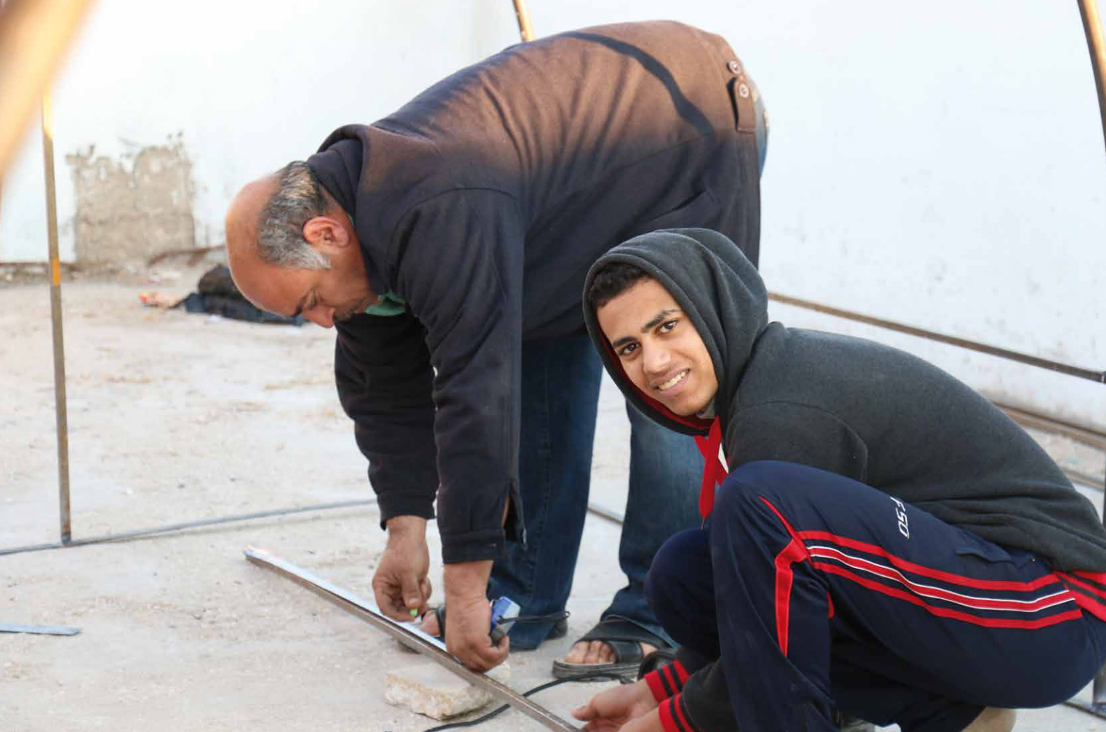
Two generations working together to create a green roof.
